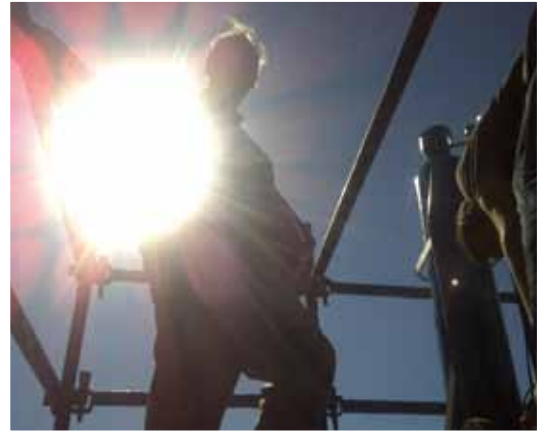
Sculptor Bruce Arnold supervises the repair to 'Our Lady'.
